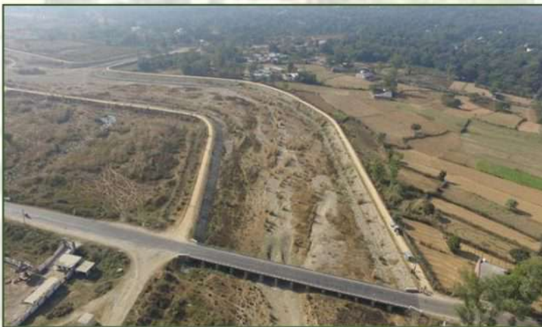
← SWAN Flood protection work, Una
